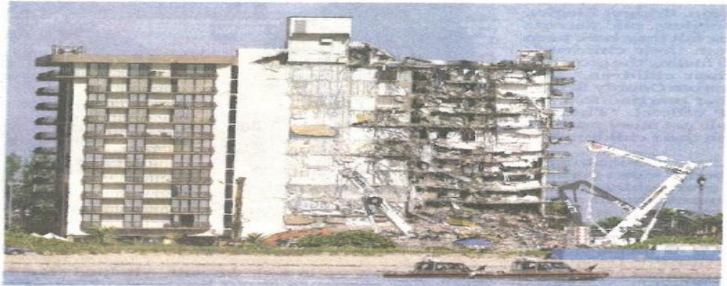
Coast Guard boats patrol in front of the partially collapsed Champlain Towers South condo building July 1 in Surfside. Champlain Towers' alarm system had been replaced in 2017. MARK HUMPHREY/AP
